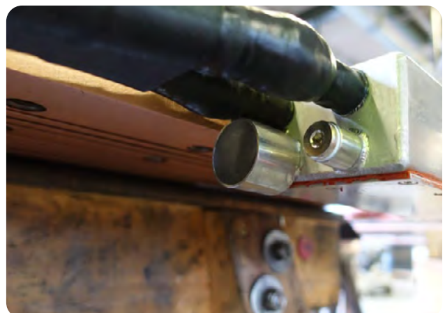
Cabling at the mould
